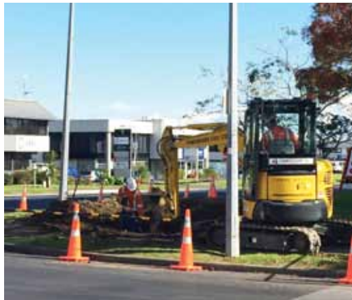
Vector power cable being replaced on Lady Ruby Drive
